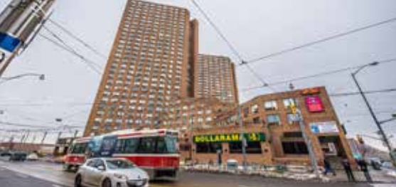
Crossways Complex Reno 77,000sq ft 2 storey addition Genreal Contractor
