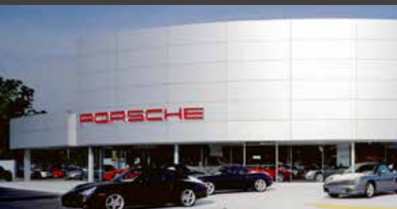
Downtown Porche Dealership 30,000sq ft Addition and Reno General Contractor
