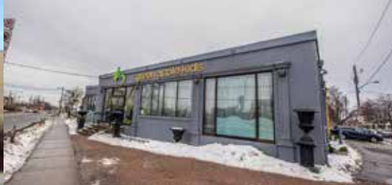
Green Apple Child Care Centre Renovations General Contractor
