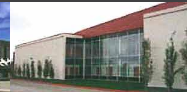
Ground Up Storage Building 120,000sq ft LEED Geo-Thermal Design/Build Contactor
