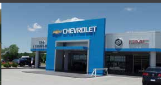
Budds' GM Dealership 30,000sq ft Addition and Reno Construction Manager
