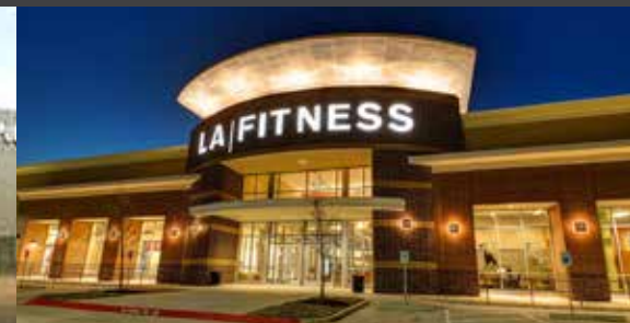
Milton LA Fitness 28,000sq ft Reno, Fitout, New Pool General Contractor
