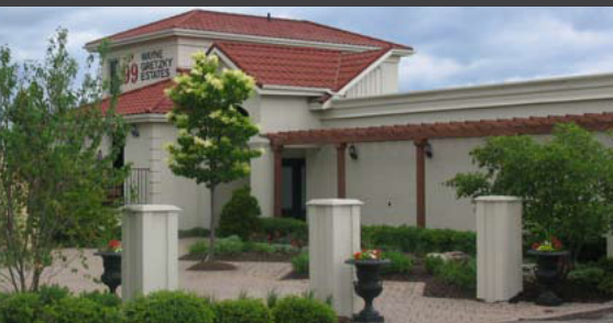
Gretsky Estate Winery Renovations General Contractor
