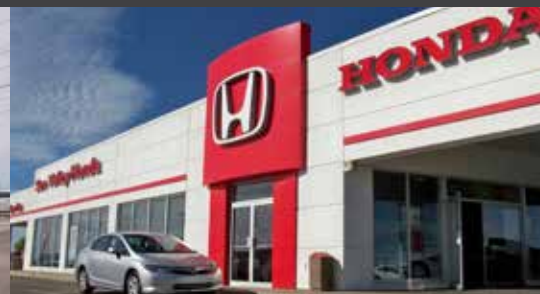
Formula Honda Dealership Interior Reno to Sales, Service, Parts General Contractor
