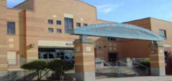
Mount Carmel Catholic High School Renovations General Contractor
