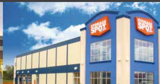
Oakville Storage Spot - 112,000 sq ft, 3-storey, ground up construction with 12,000sq ft retail plaza and restaurant pad - Design Build Contractor
