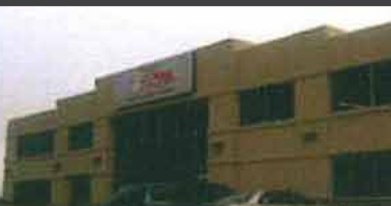
Martino Bro's Head Office 24,000 sq ft, 2 storey, Interior fitout Design/Build Contractor
