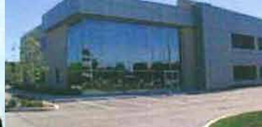
Ground Up Office and Fitout 22,500 sq ft 2 storey with parking General Contractor
