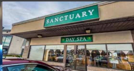
Sanctuary Health Spa Fitout and Renovations General Contractor
