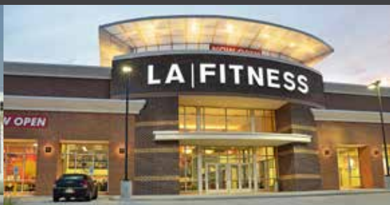
London LA Fitness 24,000sq ft Reno and Fitout General Contractor
