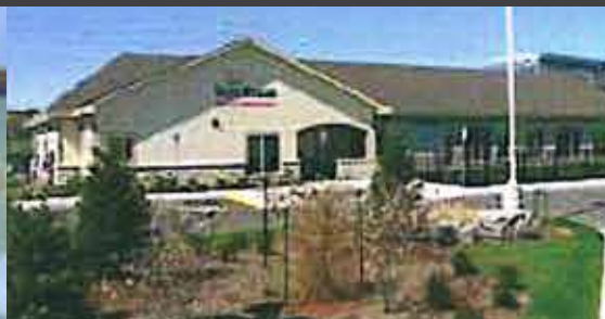
Ground Up Child Care Centre 12,600sq ft commercial kitchen General Contractor
