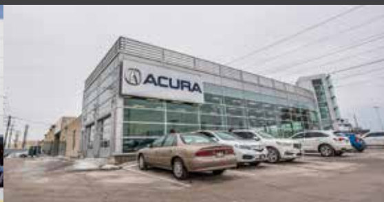
Sherway Acura Dealership 20,000sq ft Addition and Reno General Contractor
