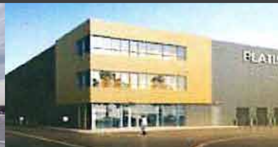
Platinum Self Storage 126,000sq ft, 3-storey, ground up construction Design Build Contractor
